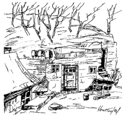
Fig. 6 The rock dwelling and cellar cut into tuff-sandstones (© V. Konečný).
